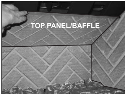
Figure 8.18 Install top panel/baffle. If rear venting, set the damper prior to installing top panel/baffle. Holding panel at an angle, place one end on top of side panel and lift other end into place. Move left or right until centered.
